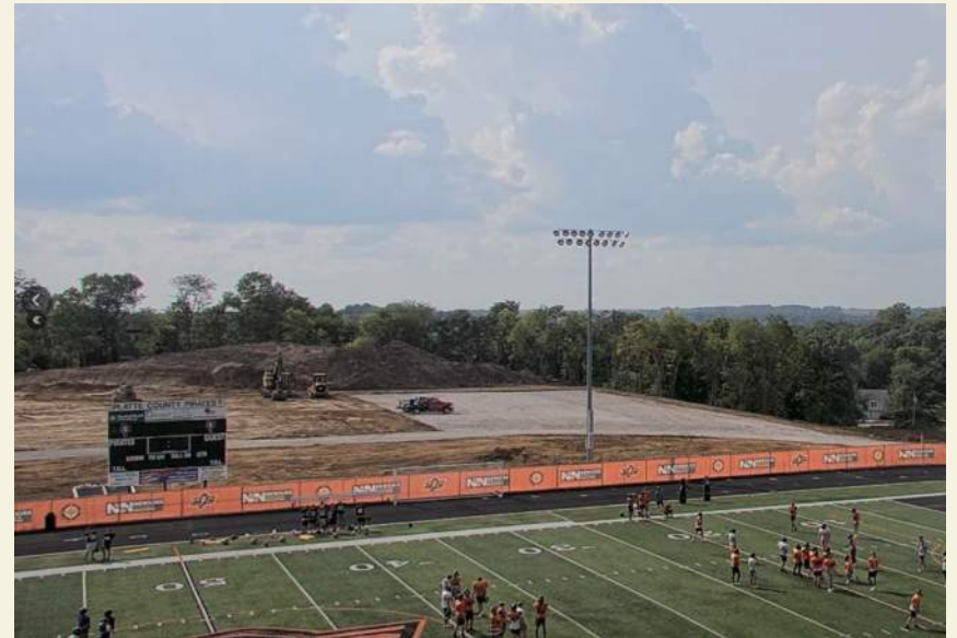
Access Road & Temporary Parking / Future Sports Practice Field
