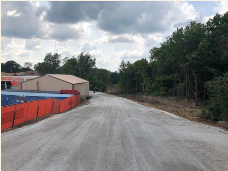
Construction Entrance / Access Road
