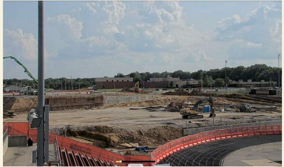
Building Construction - Walls, Footings, Site Utilities
