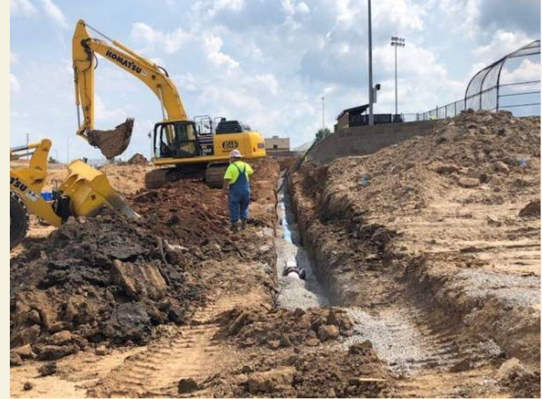
Water Main Extension
