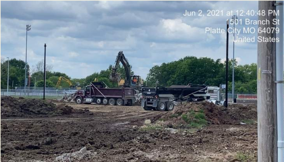
Demolition Debris Removal
