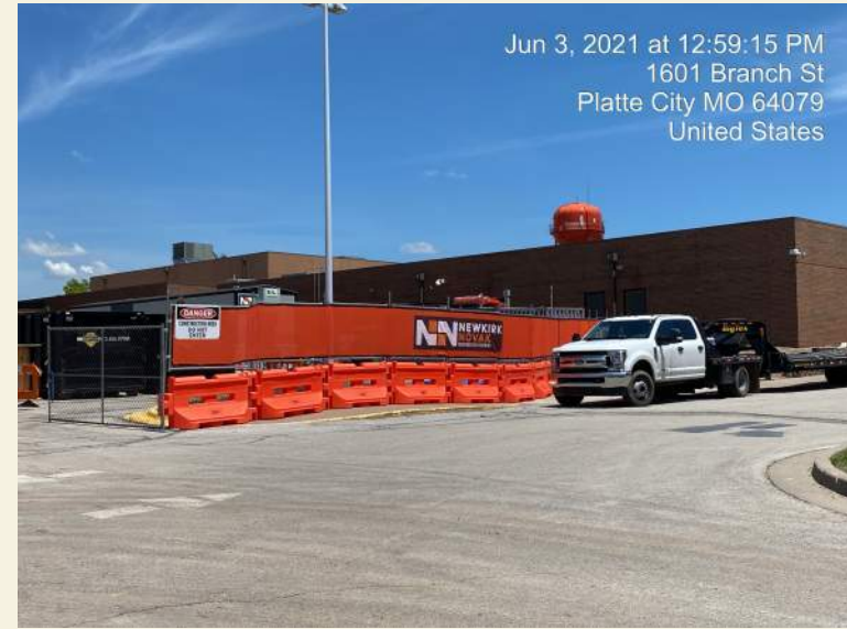
Safety Signs and Fencing Underway
