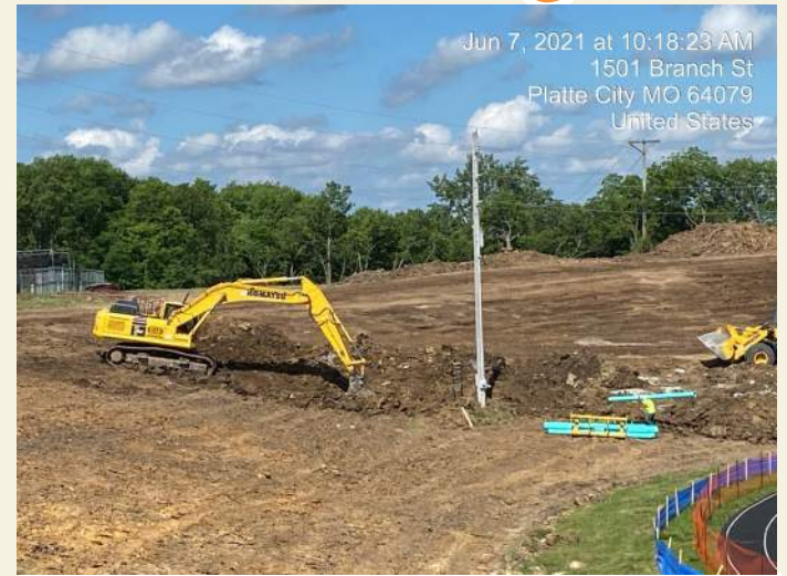
Sanitary Sewer Line Underway
