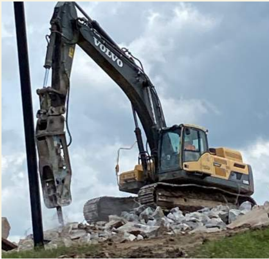
Demolition of Existing Baseball Field
