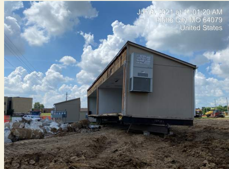
Temporary Classroom Removal
